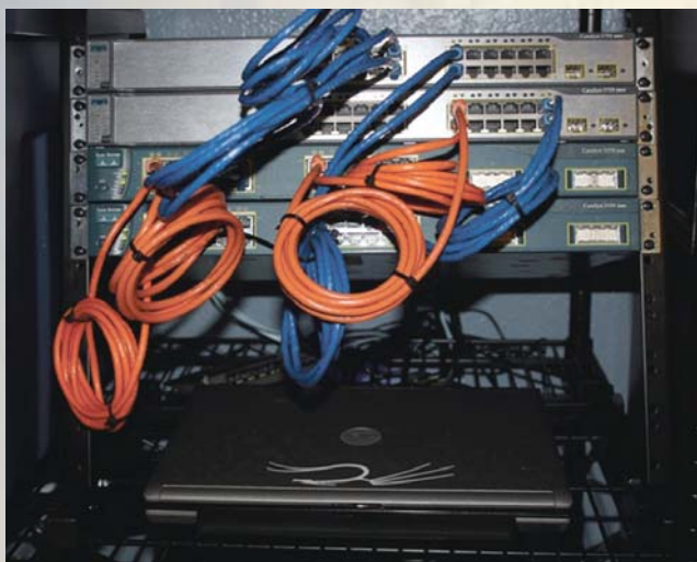
Figure 1 - Network Stack Rack for the institutions routers and network connectivity.
